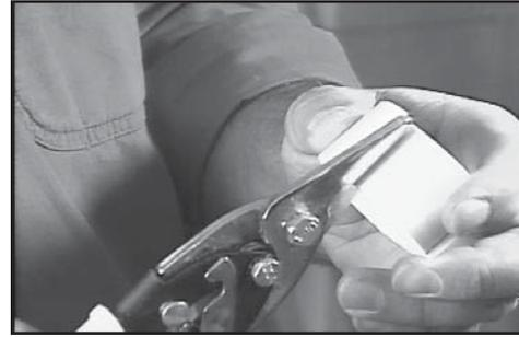
**Hint: Create clamps from extra tubing to hold low-voltage wire in place.**
